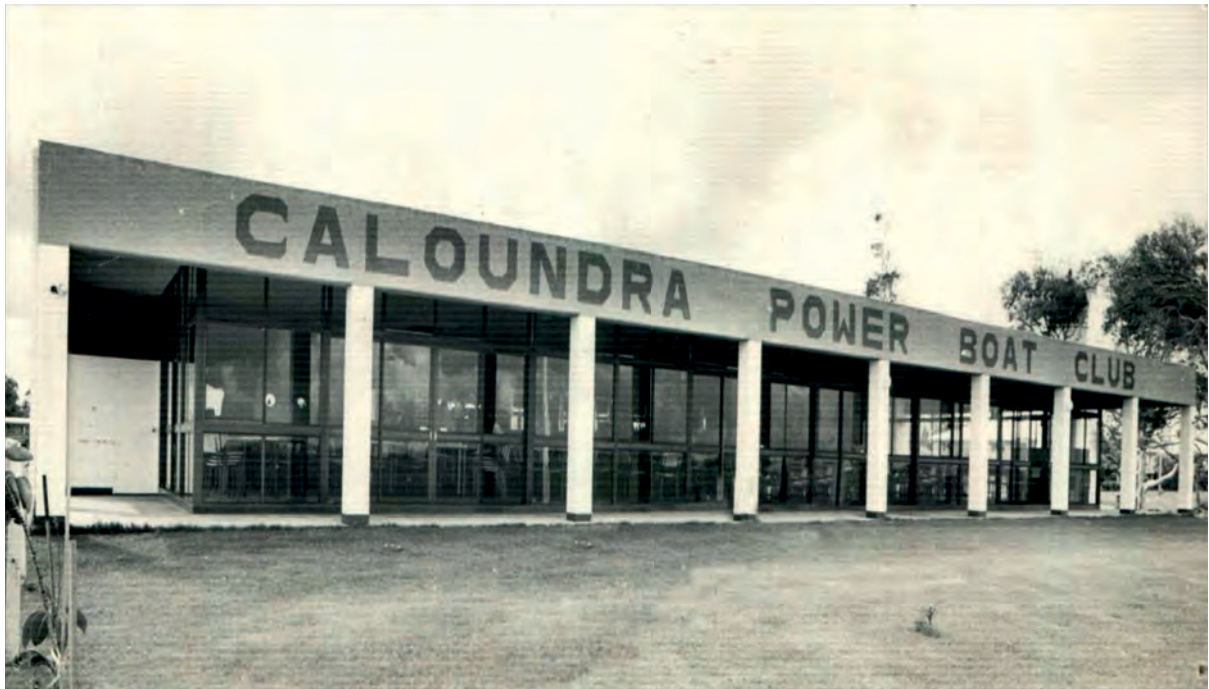
The Caloundra Power Boat Club opened a single storey building in 1978, with a concrete roof that was capable of taking additional floors in the future.
